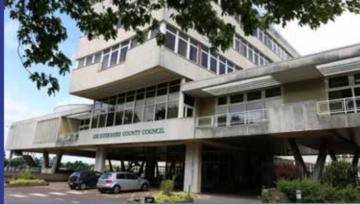
Leicestershire County Council building
